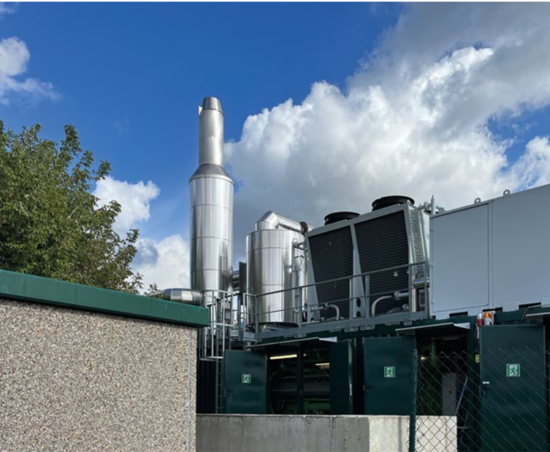
Jenbacher 320 from AB Energy Container placement
